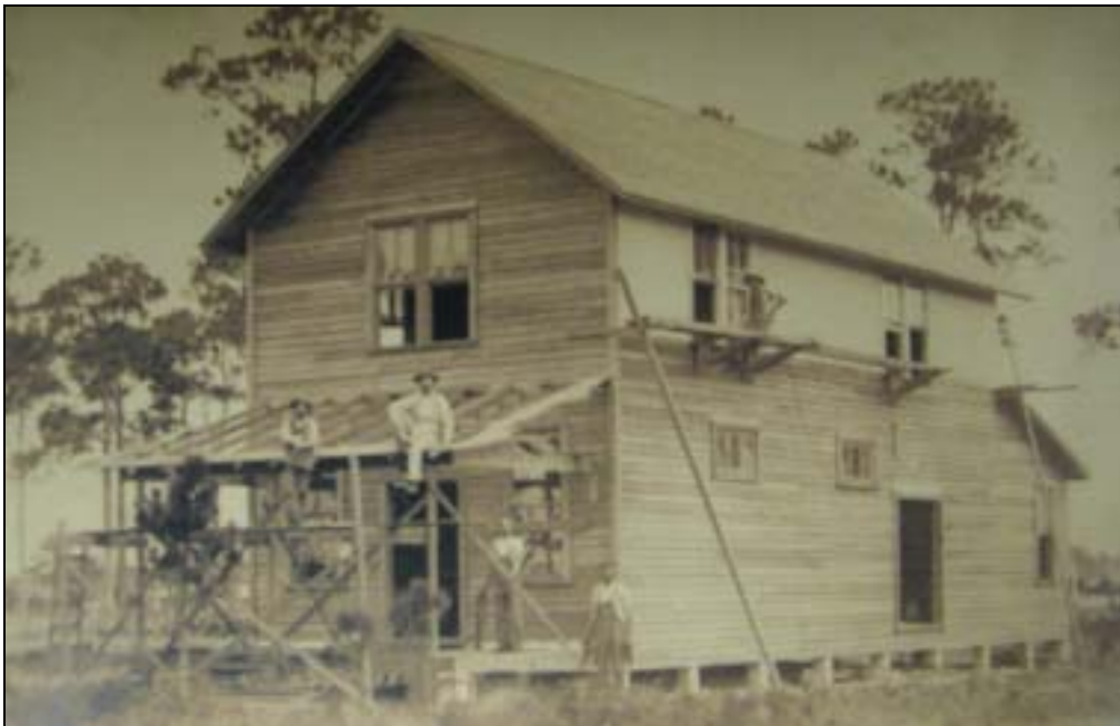
Figure 14: Construction of the White City Mercantile Building, Circa 1900 Courtesy of Mrs. Clara Sogaart LePore
