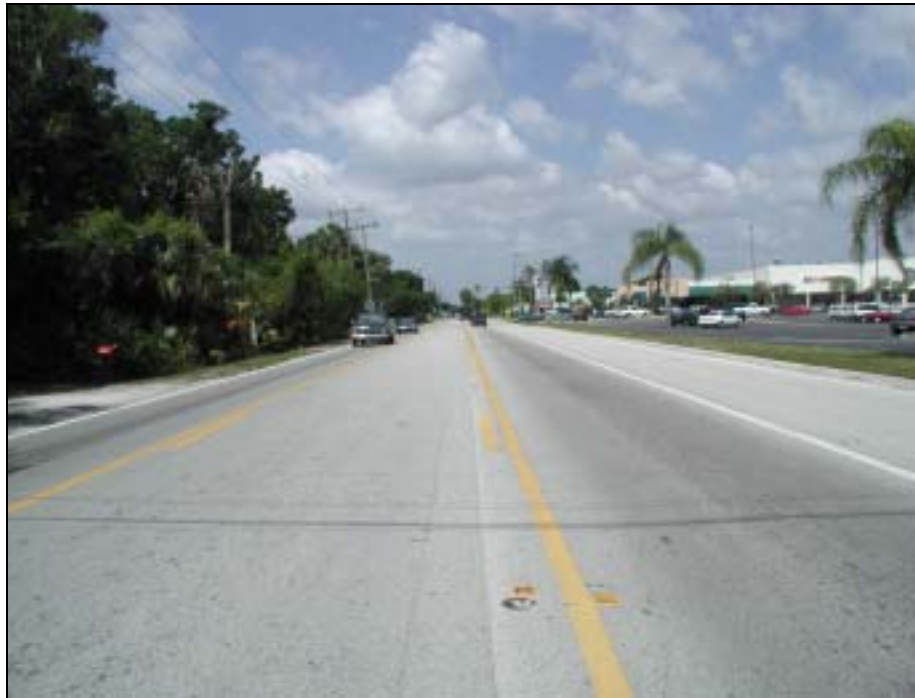
Figure 120: Midway Road just West of the Intersection of U.S. 1, Facing West
