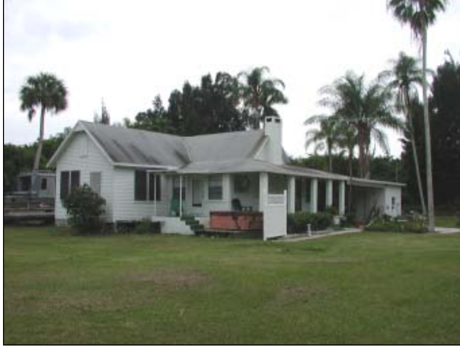
Figure 100: Current Photograph of the Shore House/Old Dixie Highway, Facing Southwest
