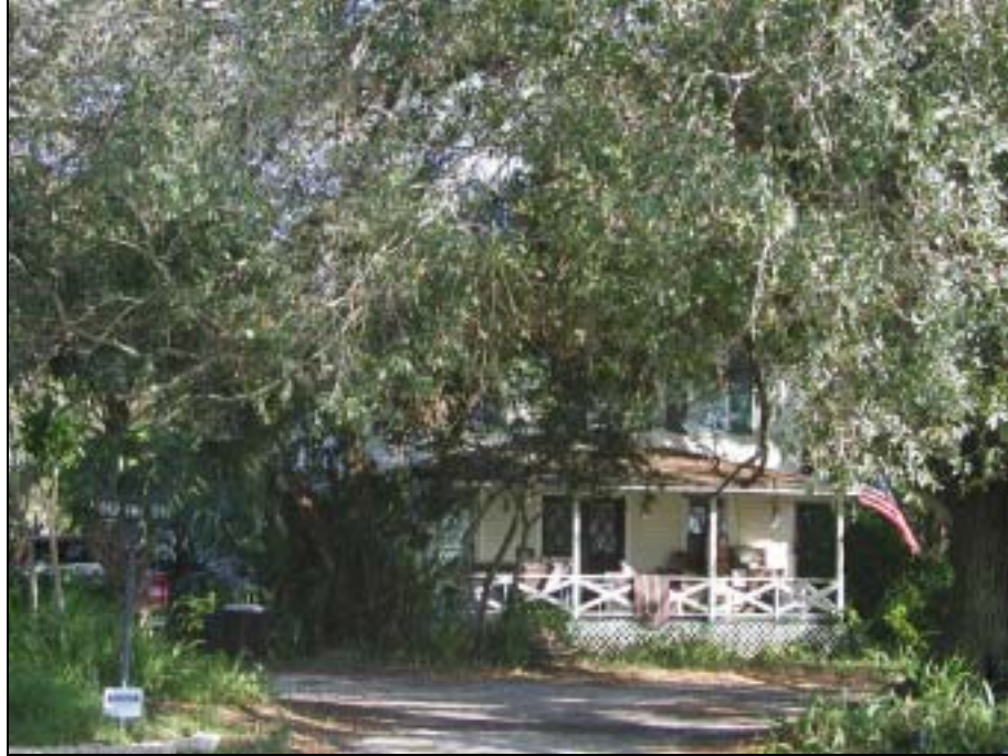
Figure 58: Pete Robinson House/5902 South Oleander Avenue, Facing East
