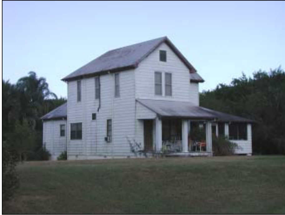
Figure 48: Keystone Grove/2950 Coolidge Road, Facing Northeast
