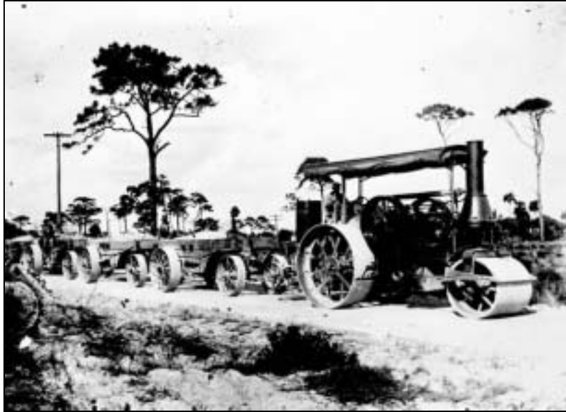
Figure 7: Construction of U.S. Highway 1 near Fort Pierce, Circa 1920
