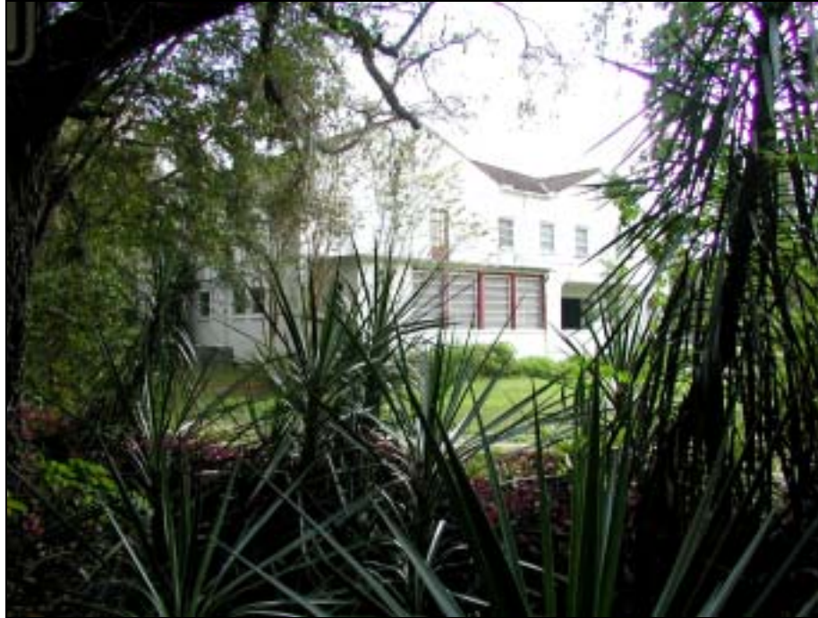
Figure 39: West (Rear) Elevation of the Binney Estate, Facing Southeast
