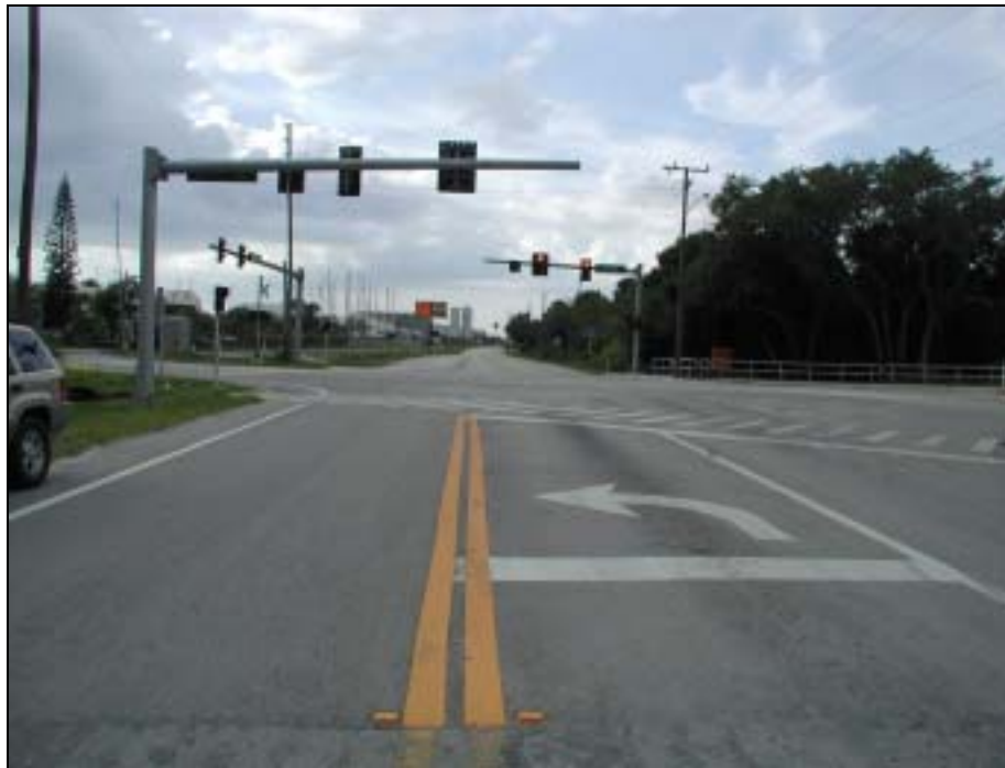
Figure 128: Dixie Highway at the Intersection of A1A, Facing South
