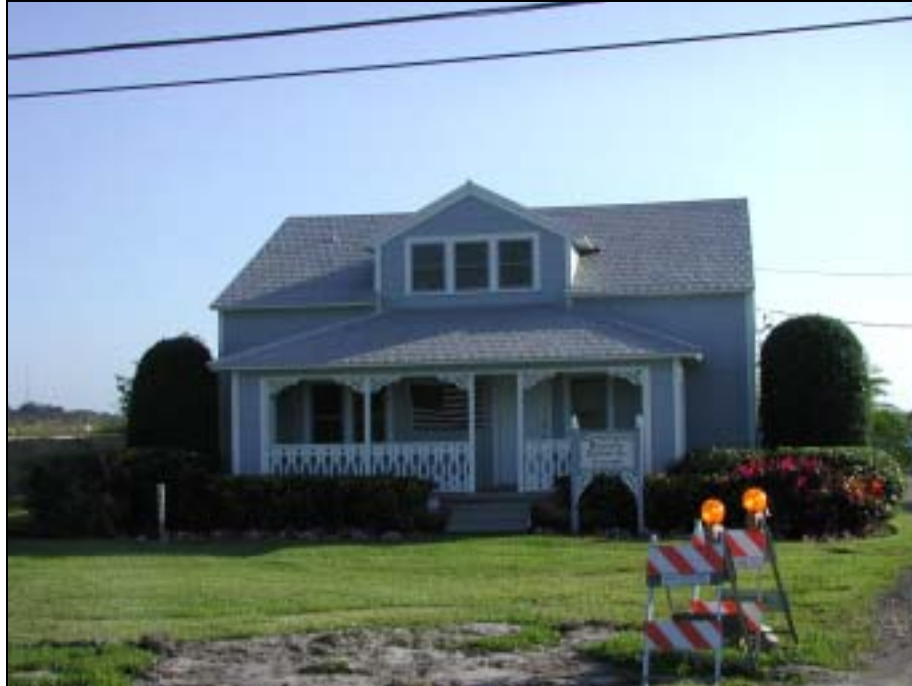
Figure 79: Counseling & Recovery Center, Inc./4753 Orange Avenue, Facing South
