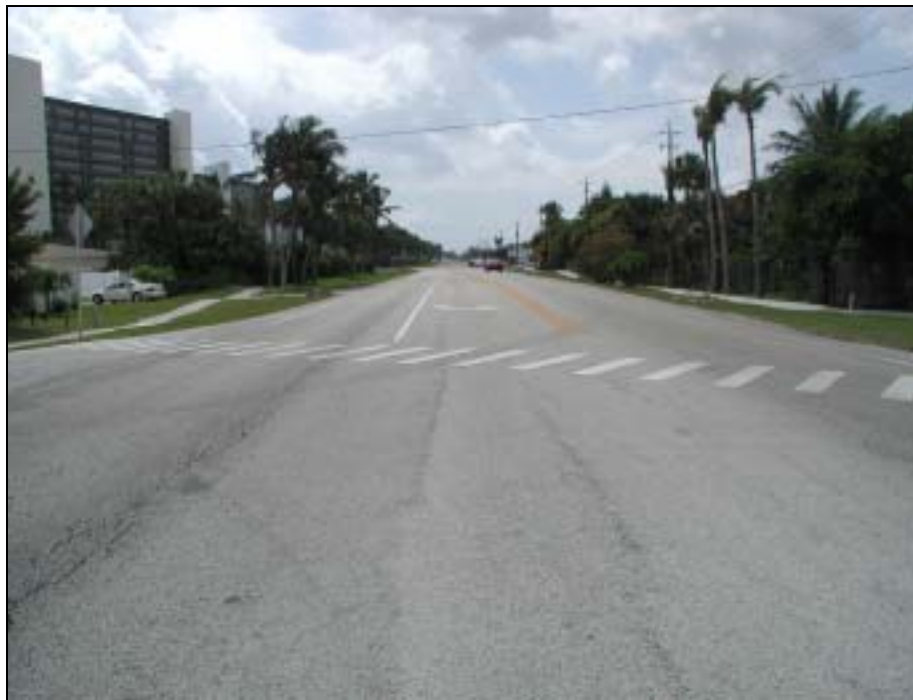
Figure 110: A1A, Intersection of A1A and Pepper Lane, Facing South
