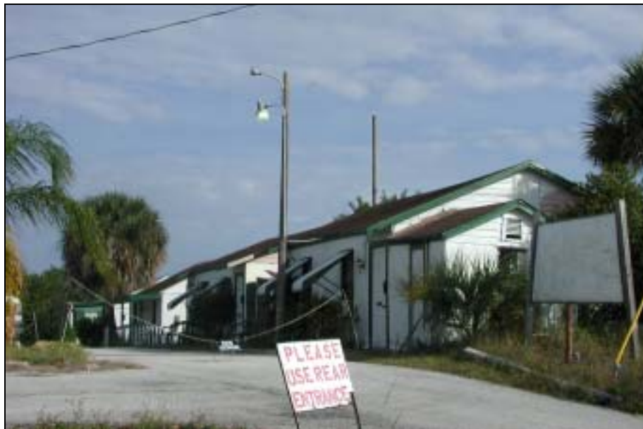
Figure 82: Wood Cottages Associated with the Dixie Summerlin House, Facing East
