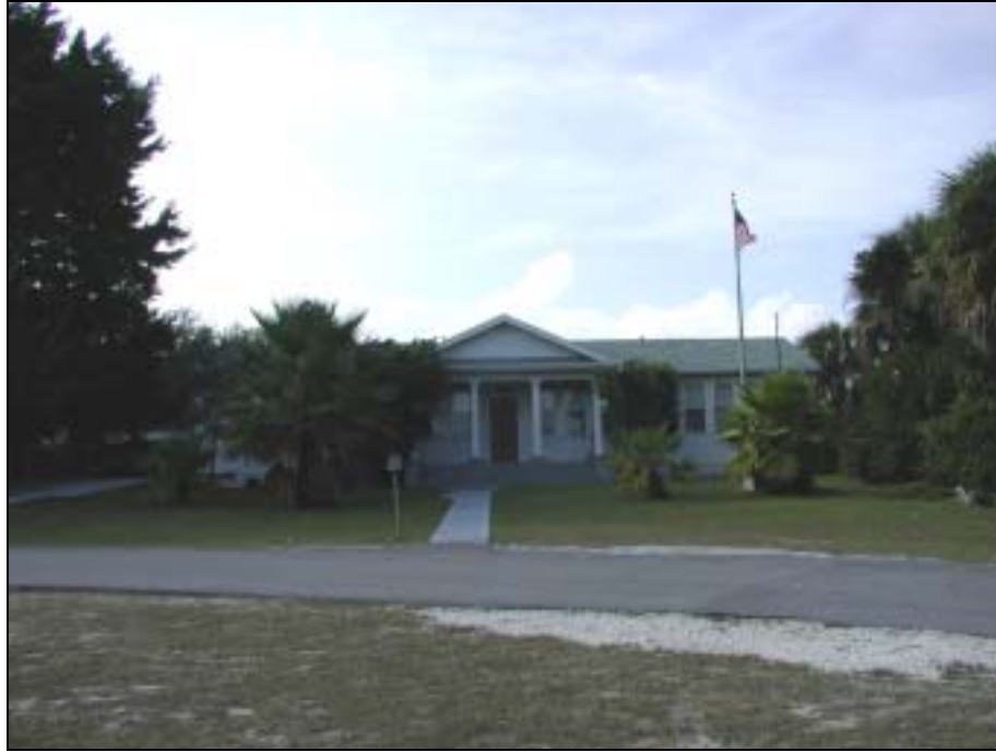
Figure 98: St. Lucie School/2501 Old Dixie Highway, Facing West
