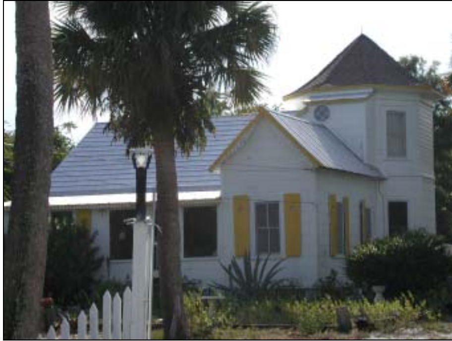
Figure 27: Example of a Folk Victorian Style Building, Located at 11995 South Indian River Drive
