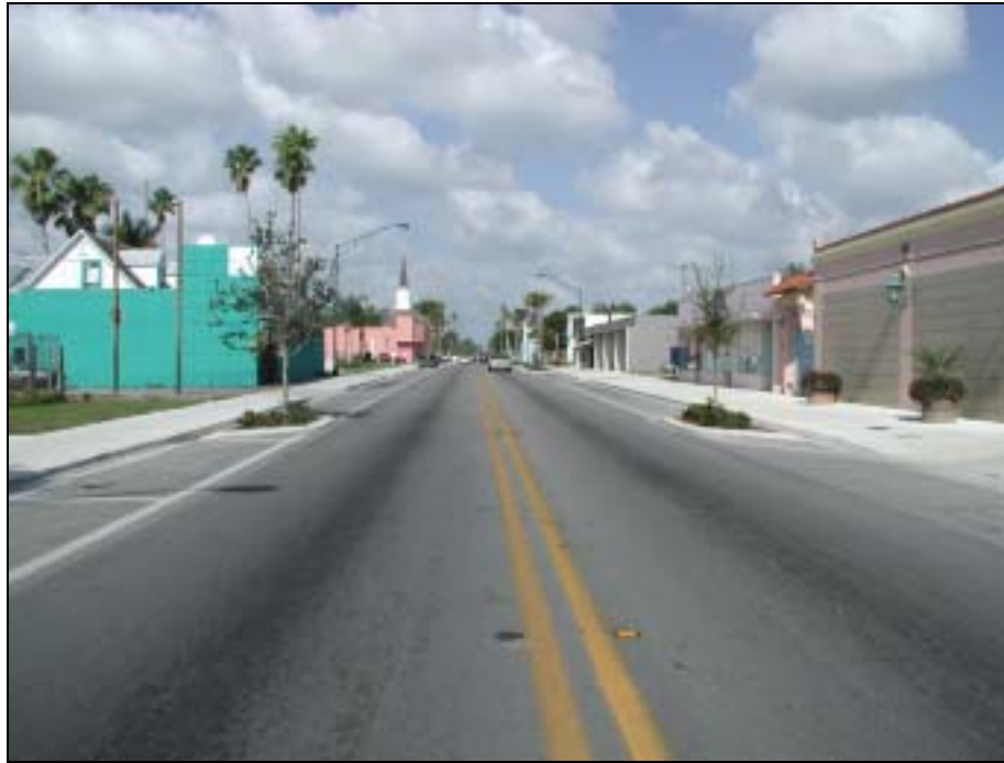
Figure 125: Orange Avenue at 7 th Street, Facing West
