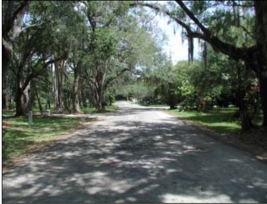
Figure 122: Palmetto Avenue, North of 1 st Street, Facing North
