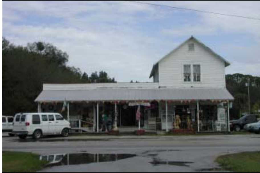
Figure 55: Current Photograph of the White City Mercantile Building/1000 West Midway Road, Facing North
