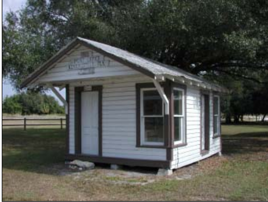
Figure 76: Kenansville Post Office/25999 Orange Avenue, Facing Northeast
