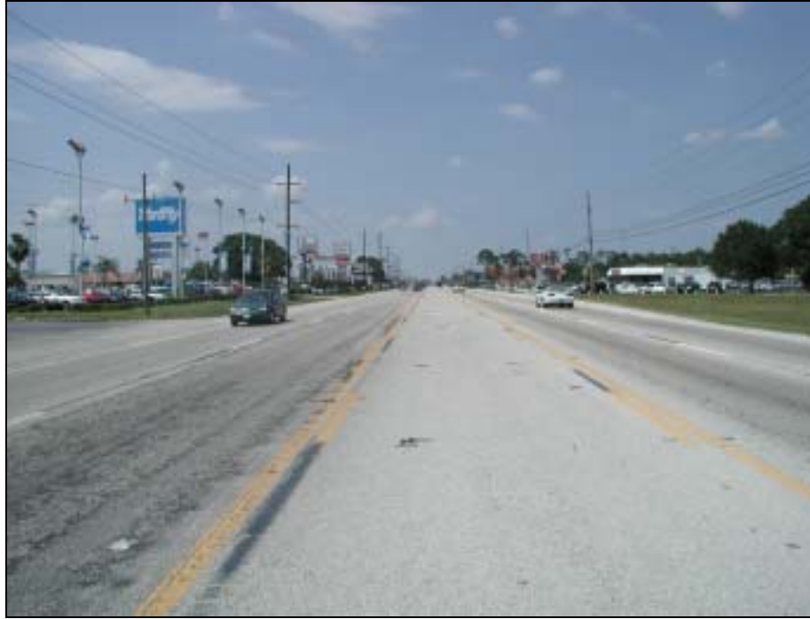
Figure 111: U.S. Highway 1 at Ulrich Road, Facing North
