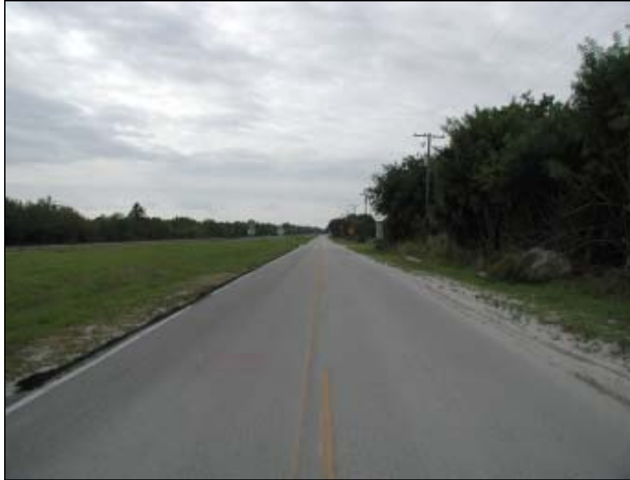
Figure 127: Dixie Highway, South of Indrio Road, Facing South
