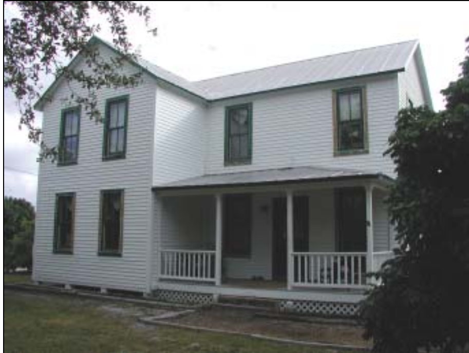
Figure 59: Nels Hansen House/5102 South Oleander Avenue, Facing Northeast
