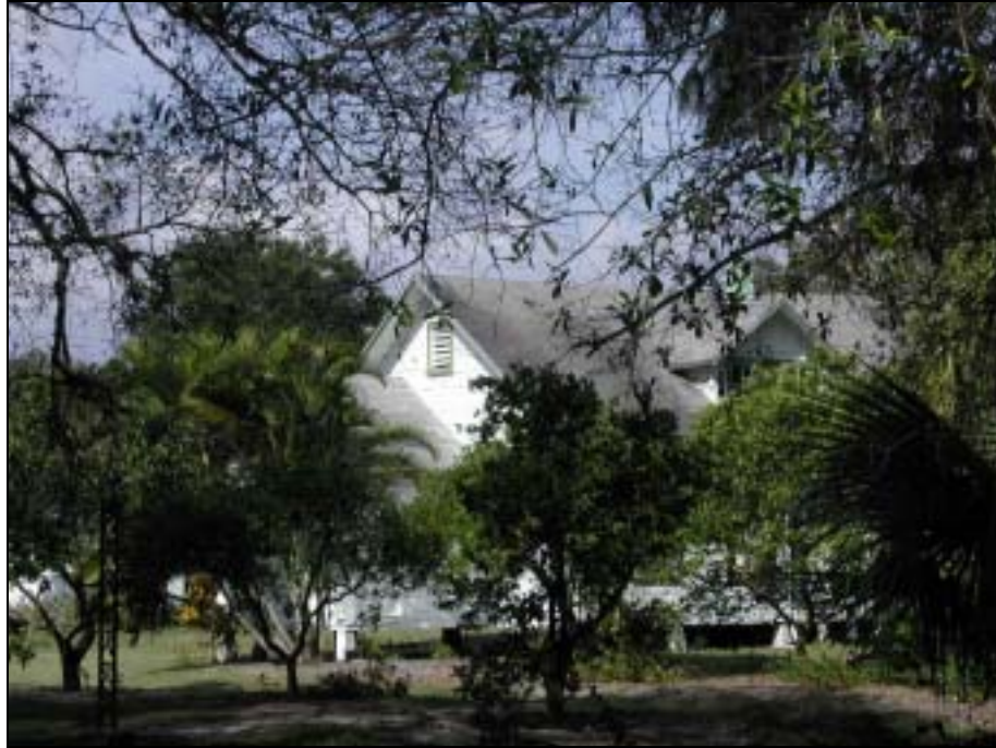
Figure 60: East (Front) and South Elevations of 4111 South Oleander Avenue, Obscured by Vegetation, Facing Northwest
