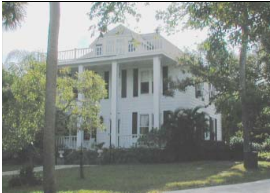
Figure 32: Example of a Neo-Classical Revival Style Residence, the R. V. Ankeny House, Located at 8205 South Indian River Drive
