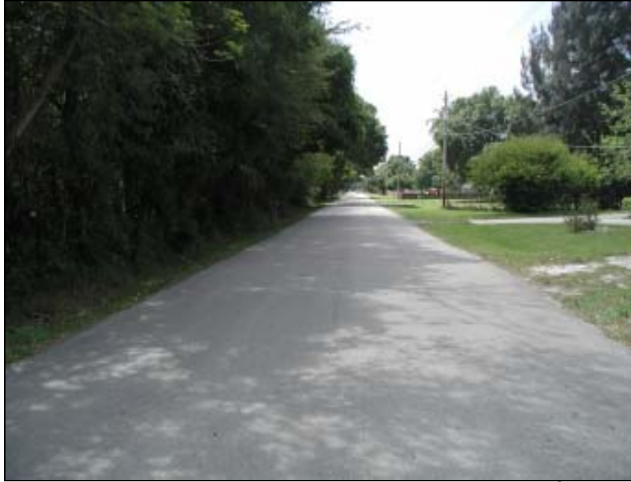
Figure 115: Citrus Avenue near the Intersection of 2 nd Street, Facing South
