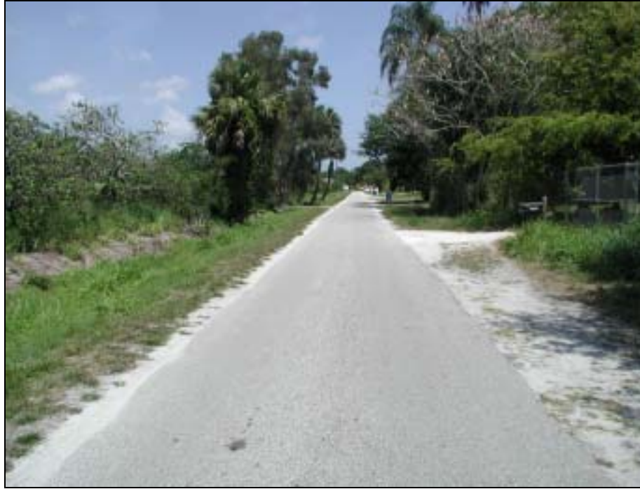
Figure 117: Approximately 4650 Elm Avenue, Facing North
