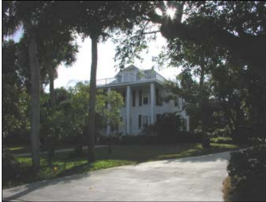
Figure 70: Ankeny House/8205 South Indian River Drive, Facing Southwest
