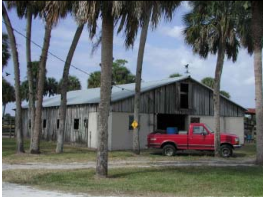
Figure 75: Wood Barn on the Adams Ranch, Facing West
