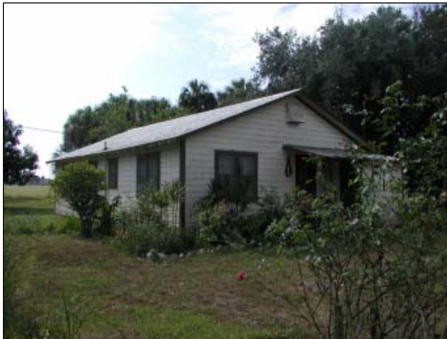
Figure 74: Frame Vernacular Residence on the Adams Ranch, Facing Southwest
