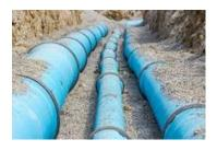
This project, consisting of 8,300 lineal feet of 16" water main and 12" force main between the Indrio Road and Emerson Avenue intersection and existing infrastructure at the Indrio Road and Taylor Dairy Road intersection and on the Turnpike Feeder Road, is phase 3 of the previously completed 2 phases associated with looping the Indrio Road, Taylor Dairy Road and US1 corridor enhancing the water flow availability and the wastewater
