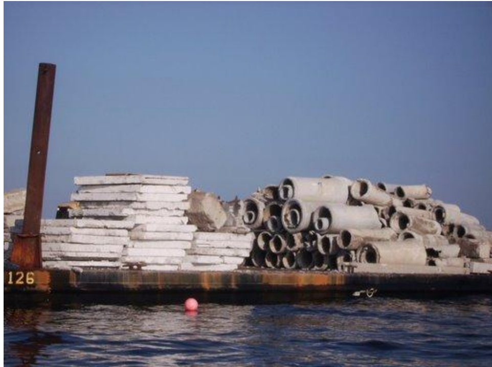
Figure 2 Barge load of materials prior to deployment 8/27/08 – slabs, culverts and large chunks.
