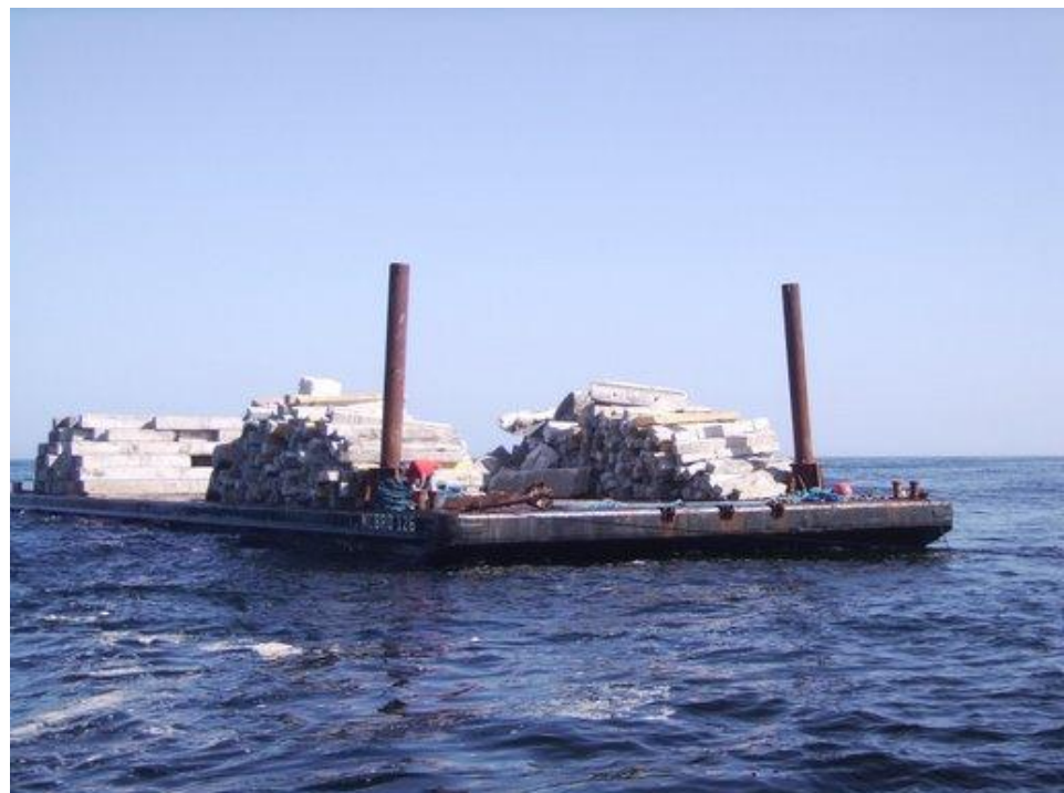
Figure 3 Barge load of materials prior to deployment 8/28/08 – piling cutoffs and RR ties).
