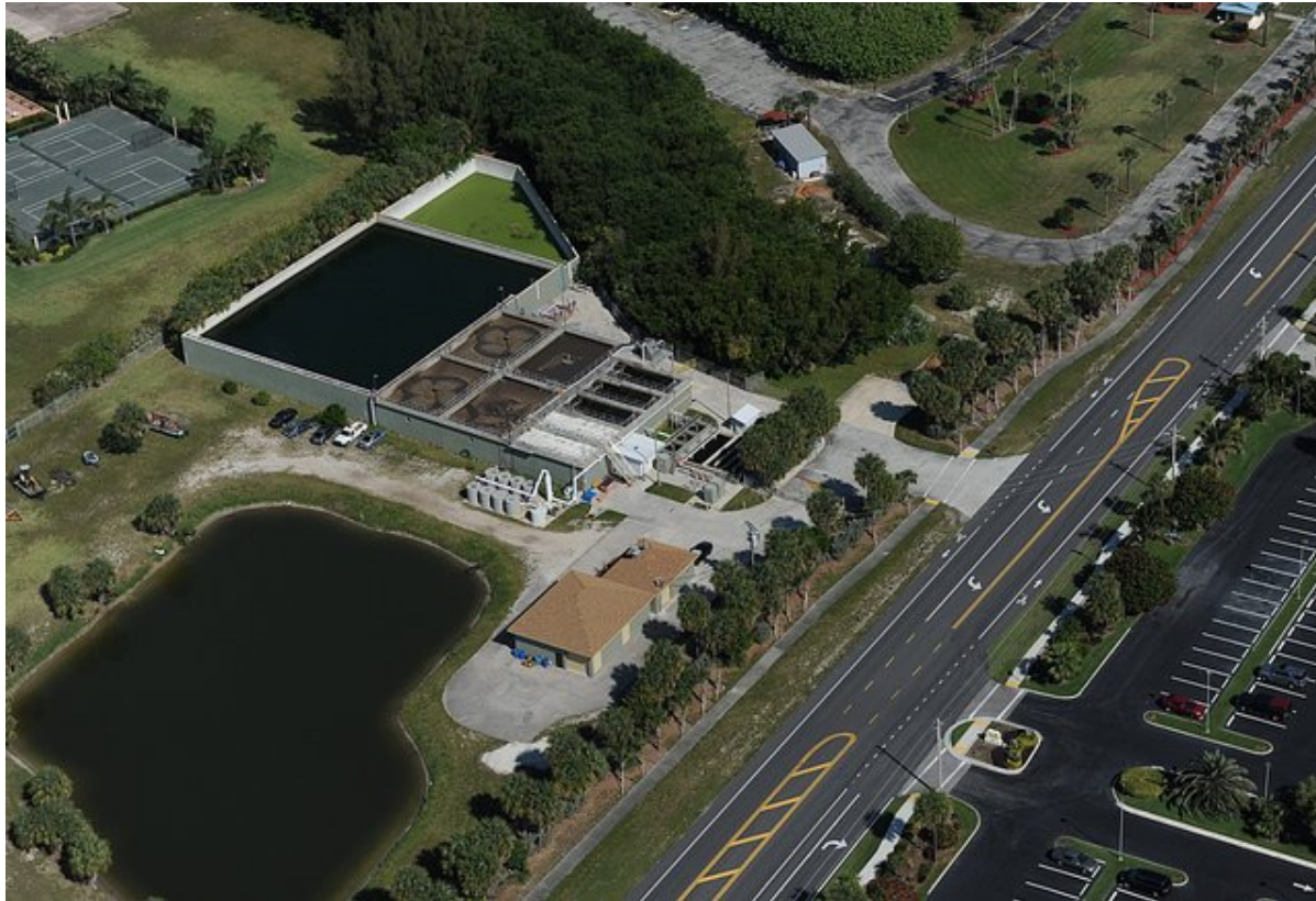
North Hutchinson Island Wastewater Treatment Plant
