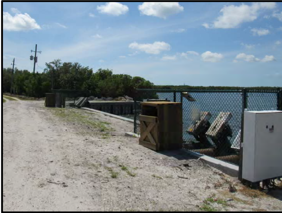
PHOTOGRAPH #02: NEW SHEET PILE WALL AFTER CONSTRUCTION, JUNE 2020
