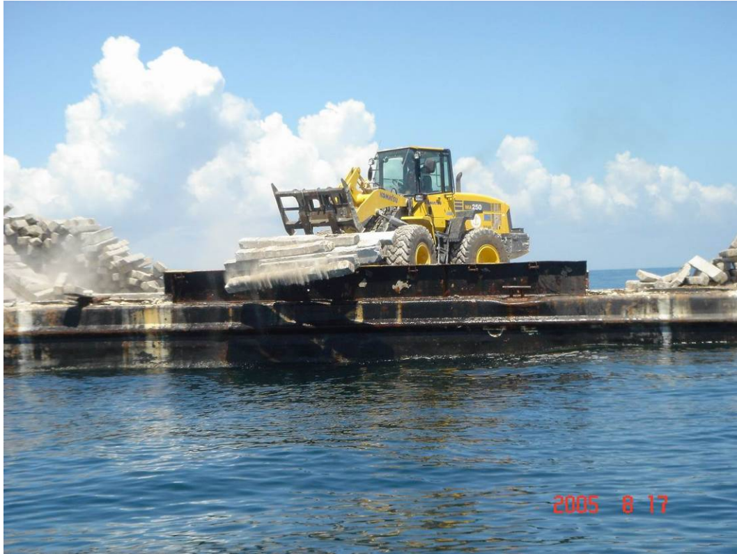
Figure 6. 2005 Photograph of Deploying RRties from Barge
